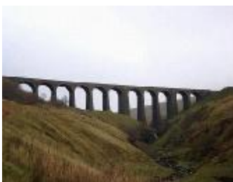
Arden Gill Viaduct, Railway Walk
